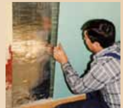
Positioning the board and fastening with screws
